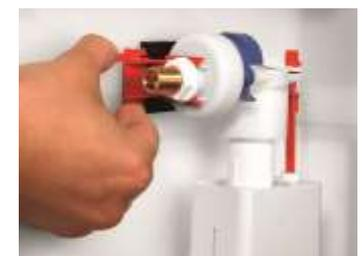
The inlet valve can now be easily removed for inspection or replacement of washers.
